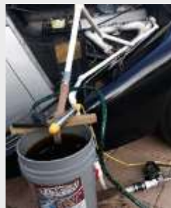
Hot Chemical Flush
